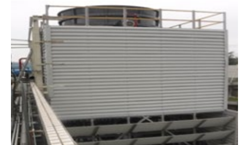
▶ 冷卻水塔汰換／擴充
